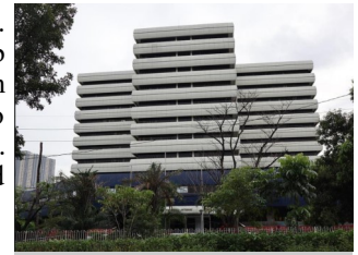
Bureau of Internal Revenue Bldg in BIR Road, Quezon City (Photo by Patrick Roque via Wikimedia Commons CC BY-SA 4.0)
